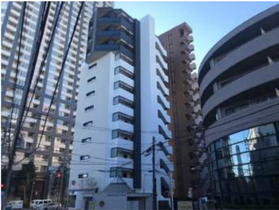
October 2018 (immediately after completion)
